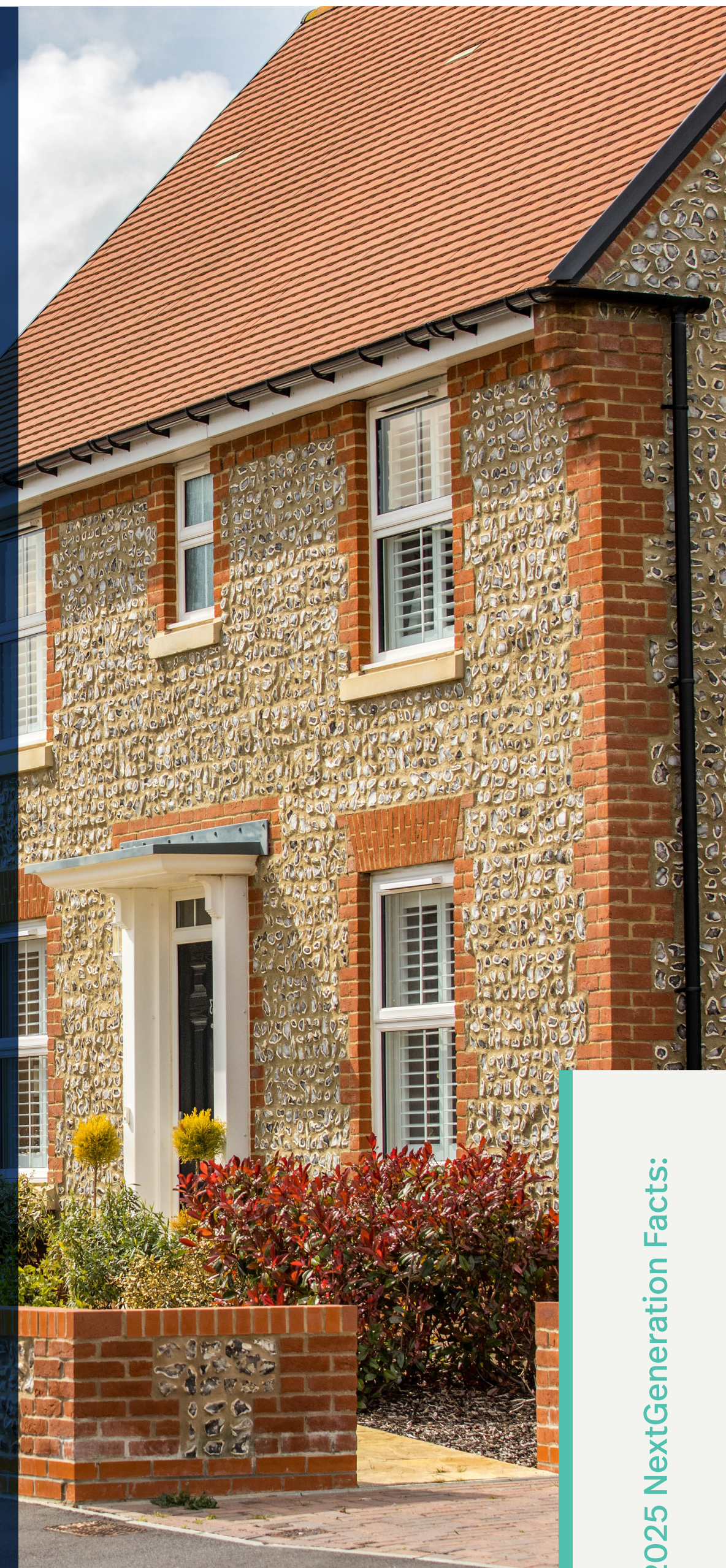
Photo courtesy of Barratt Redrow plc
